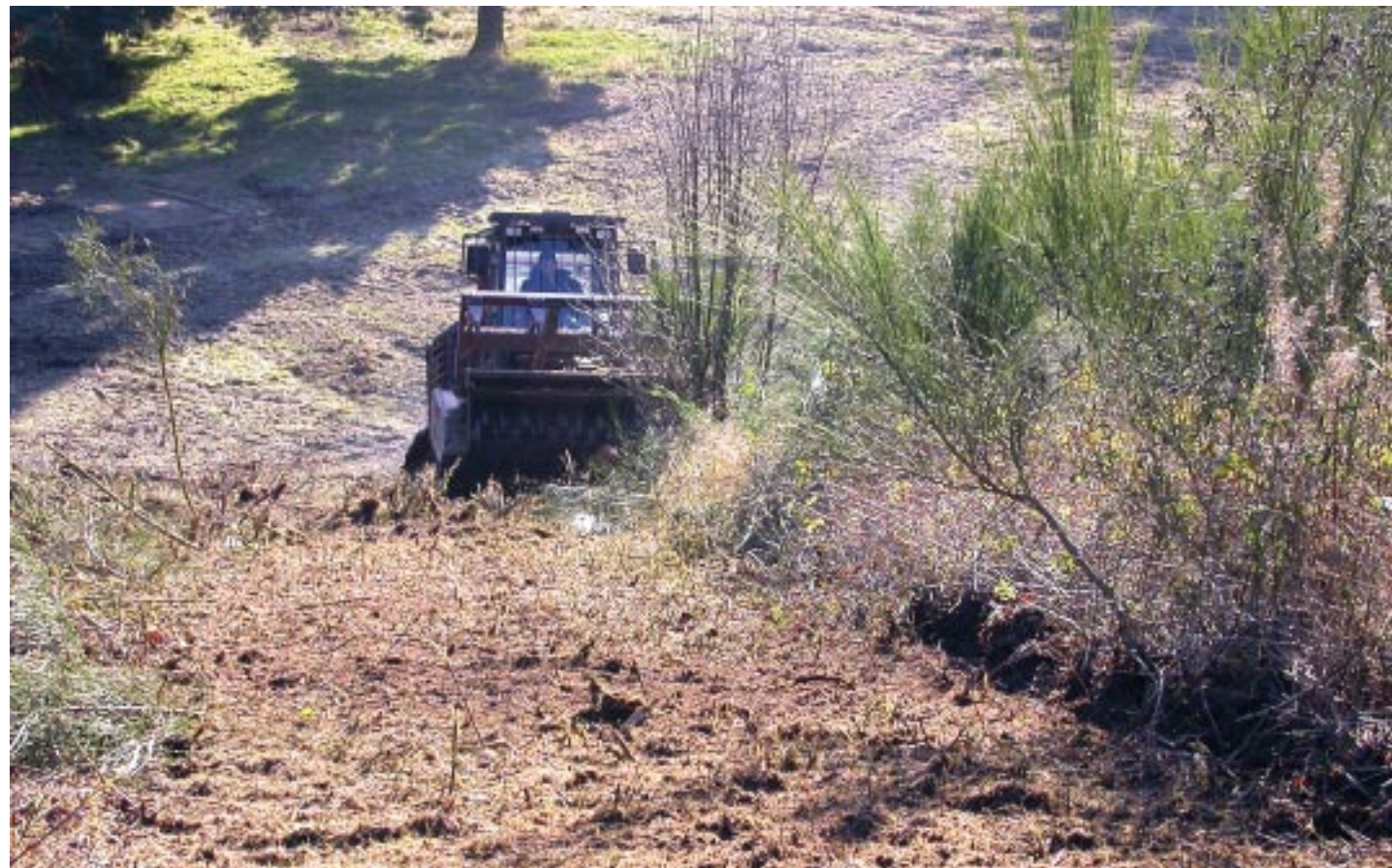
Clearing of overgrowth
