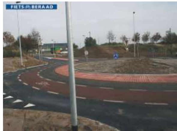
A cycle lane marked in the middle of the roundabout lane (image source: Fietsberaad)
