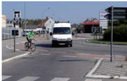
The dangers of a cycle lane on a roundabout (source: Vademecum fietsvoorzieningen – Brussels)
