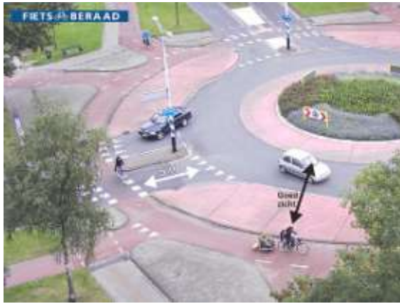
Single-lane roundabout with cycle track, with right of way for cyclists (Enschede, NL). Notice the typical circular design of the track and the colored crossings.
