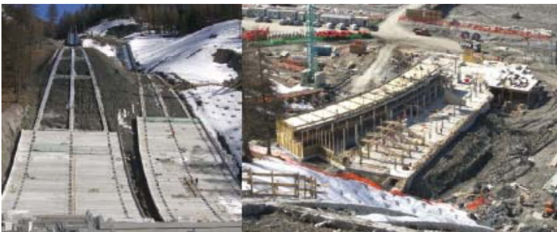
Figure 12_Ski jumping facility
