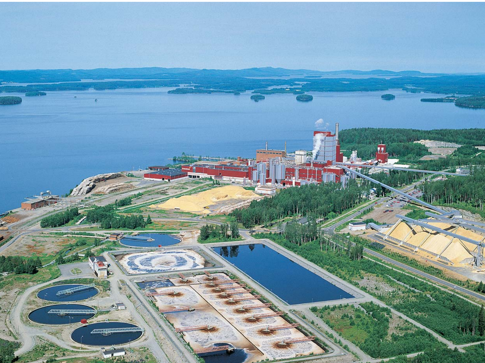
Enocell Pulp Mill. The activated sludge plant of the effluent treatment plant in the front.
