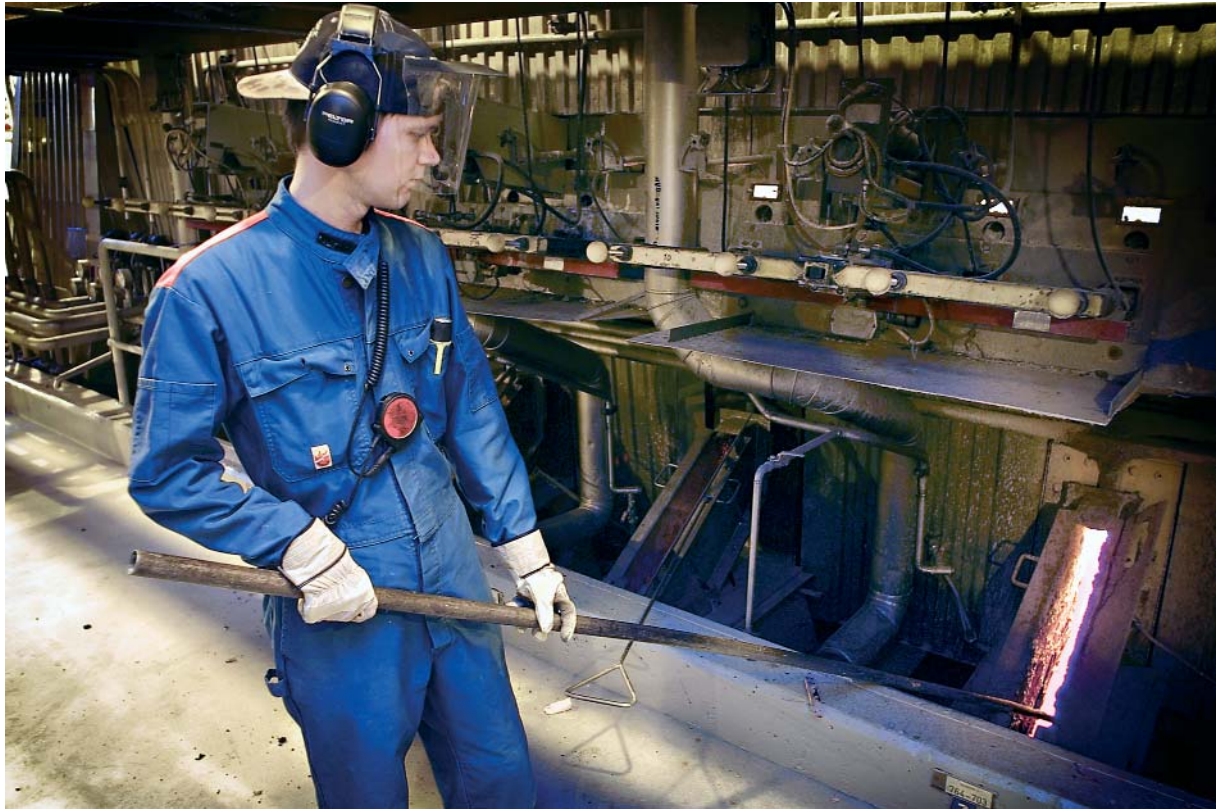
The smelt outlets of the recovery boiler are cleaned in order to guarantee even cooking.
