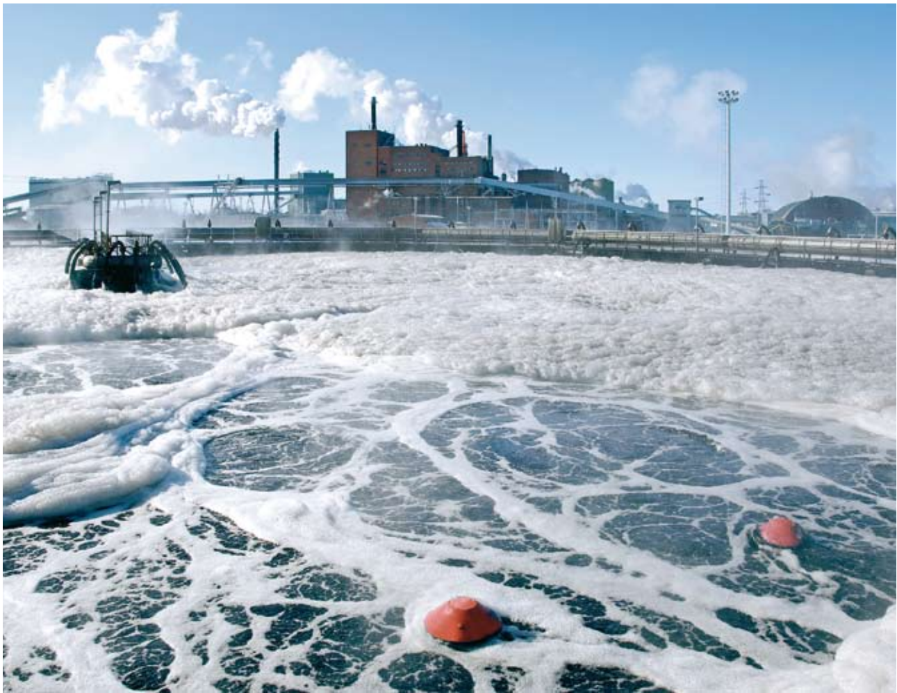
Biological wastewater treatment plant.
