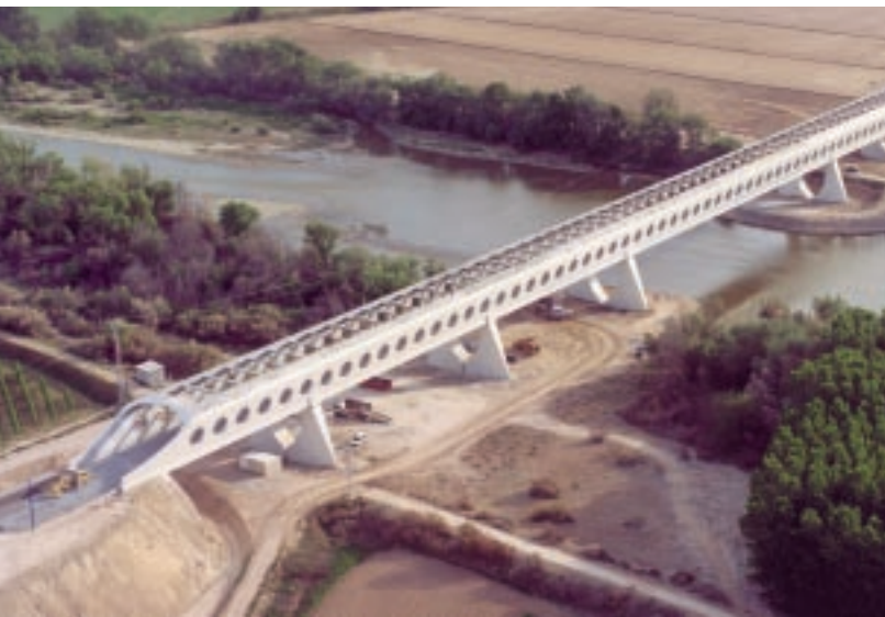
High-speed line Zaragoza–Lleida: Bridge over the Ebro river (GIF)
