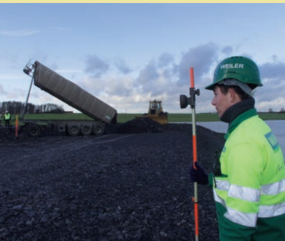
Embankment works at Baudrecourt (France) (La Vie du Rail/Michel Barberon)
