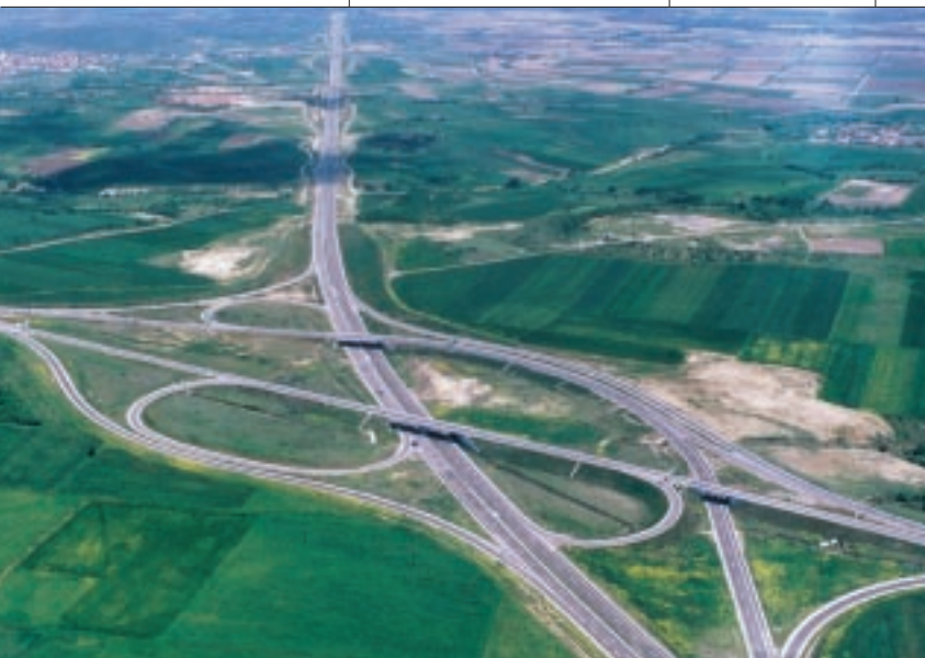
Intersection of Via Egnatia and trans-European axis IX (Egnatia Odos A.E.)
