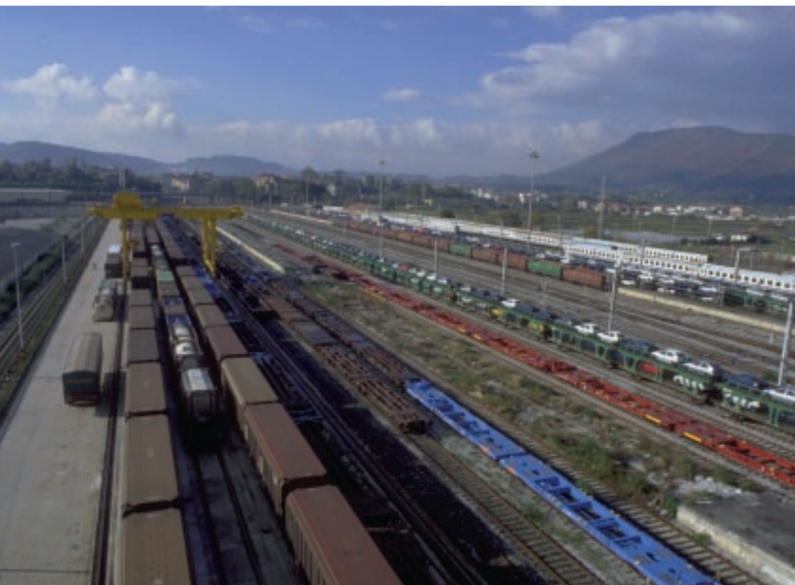
Railway yard at Playa-Aundi (Irun station) (SNCF Centre audiovisuel)
