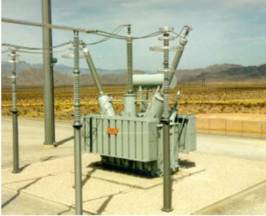
*Station de compensation 400 kV 160 MVA*
