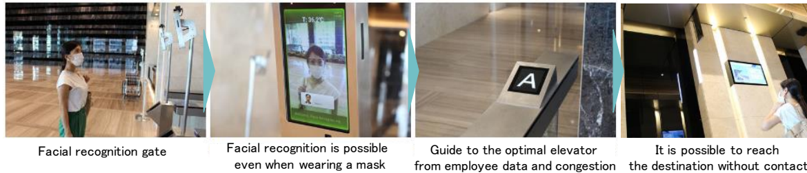
Figure 8. ELE-NAVI system linked to the facial recognition gate
