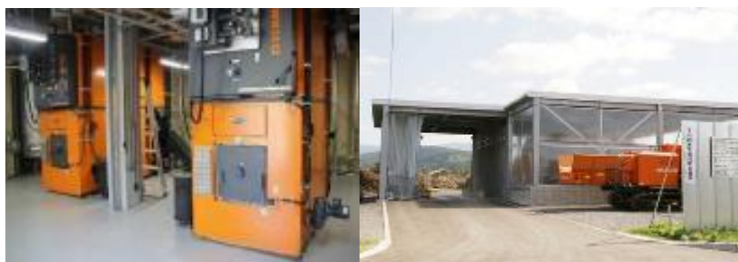
Figure 4 Wood Pellet Biomass Boiler and Pellet Manufacturing Plant
