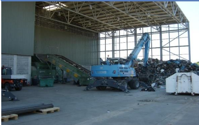
On-site crane for sorting waste in Pecs, Hungary
