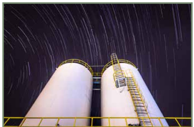
Start-rails behind dehydrated sludge silos at the Barreiro/Moita waste-water treatment plant, Portugal – Eduardo Ventura
