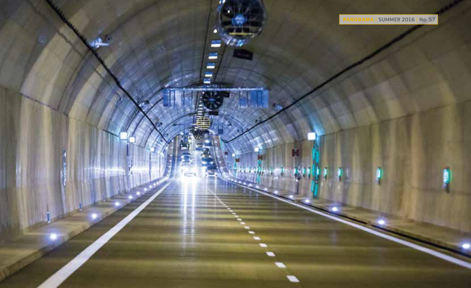
Tube tunnel below Martwa Wisła
