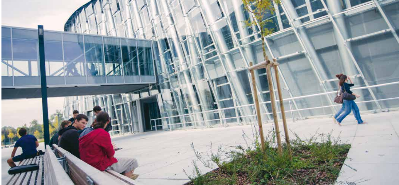
▶ LJUBLJANA, SLOVENIA: New facilities for the Faculty of Chemistry and Chemical Technology and the Faculty of Computer and Information Science have boosted capacity for natural sciences and technology research.
