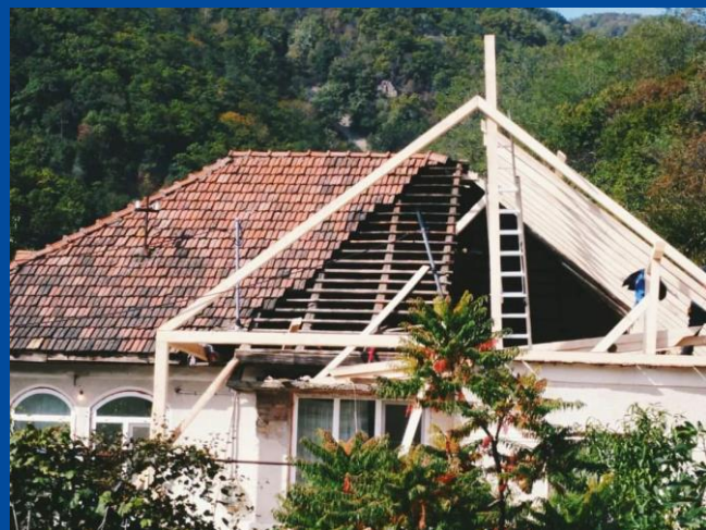
House being renovated in Bumbesti Jiu
