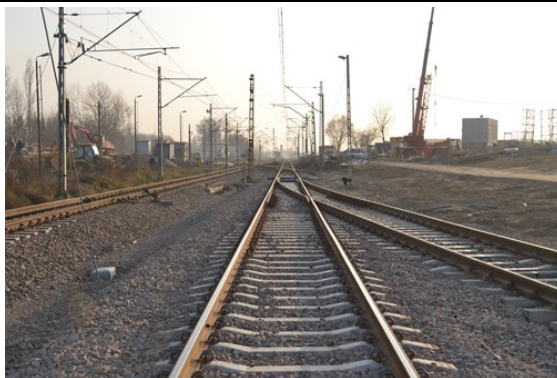
Figure 13. Modernisation of the railway track of the line no. 8
