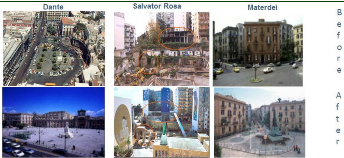
Figure 4. Examples of Urban regeneration and in the Vanvitelli–Dante segment of Metro Line 1 in Naples.
