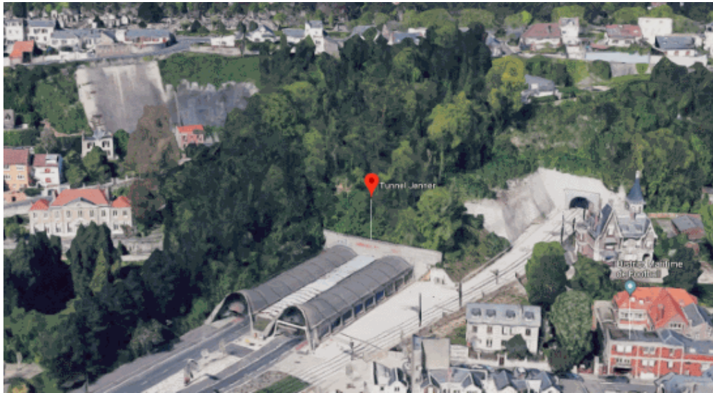
Figure 11. Lower City entrance of the Tunnel Jenner.
