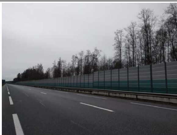
Figure 10. Noise protection walls
