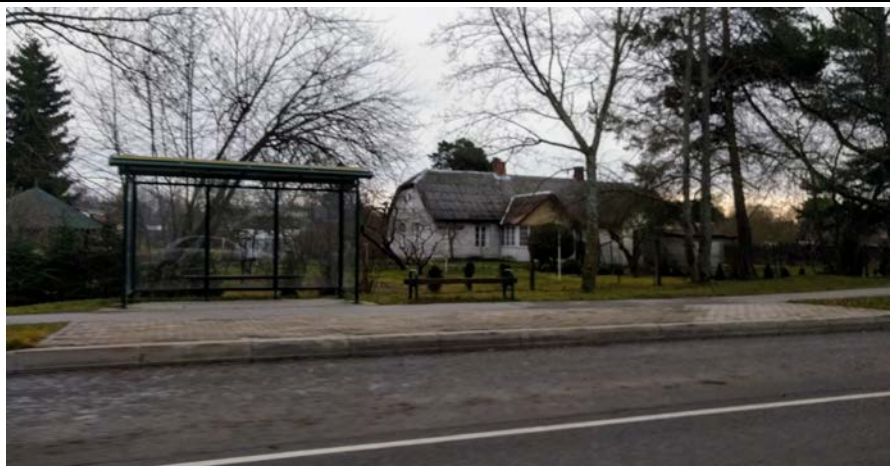
Figure 13. Reconstructed bus stop and sidewalk
