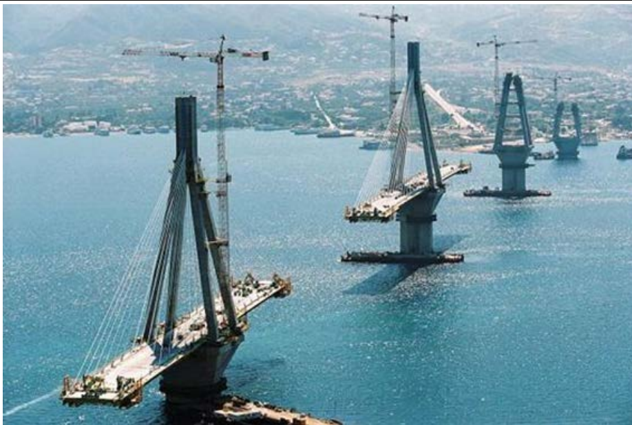
Figure 10. Rio-Antirio bridge under construction
