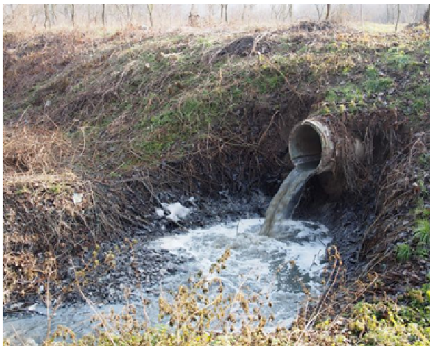
Waste water spill
