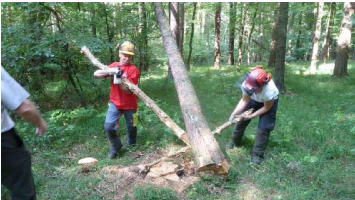
(Photo 12: ICC2 Taking down a hung-up tree with poles-Czech Republic: Robb 2011)
