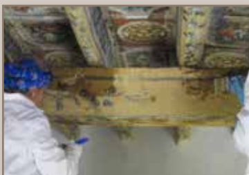
Restoration of decoration
