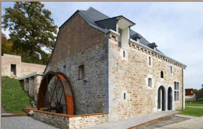
After the renovation
