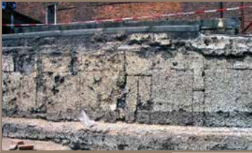
Draining the masonry
