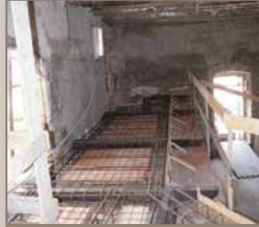
New structure in reinforced concrete
