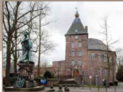
Entrance tower and Western facade (ivy already removed)
