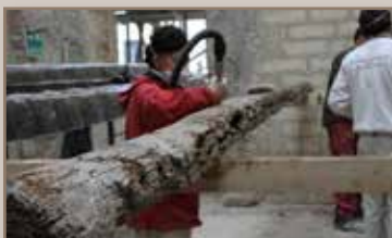
Restoration of wooden sleepers
