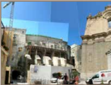
During the renovation
