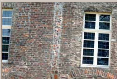
Repaired crack in the facade
