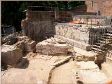
During the renovation (in front of the southern façade)
