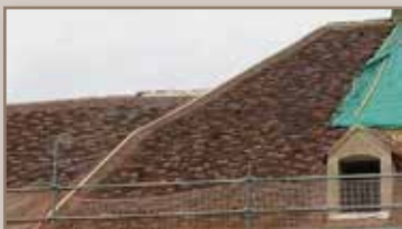
Mixing of old and new tiles and realization of the middle corner of the mansard roof
