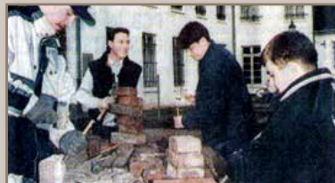
Cleaning and repairing of broken stones
