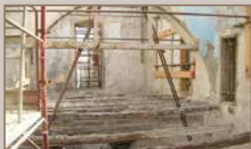
Removal of the original floor
