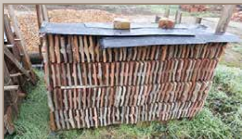
Removal and storage of the ridge tile and removal of the damaged battens and chevrons
