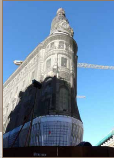
During the renovation
