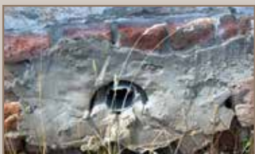
Removing old plaster
