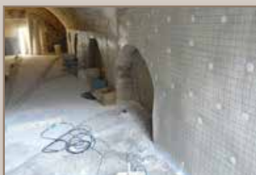
Restoration of the masonry
