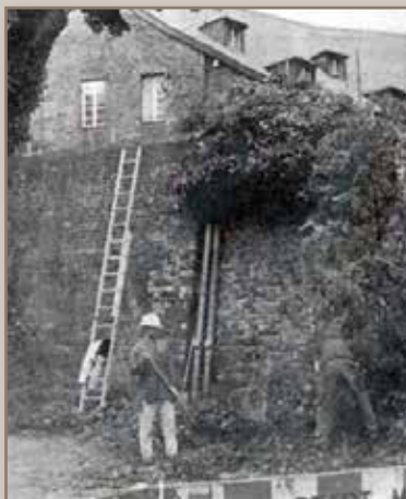
Removing plants in the masonry
