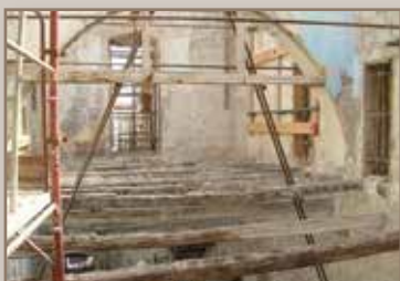
Removal of the floor
