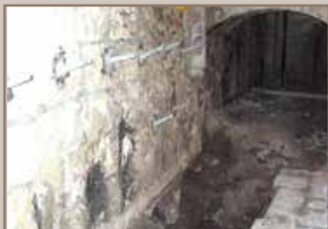
Consolidation of the walls
