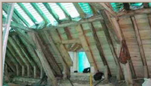
Consolidation of the frame elements
