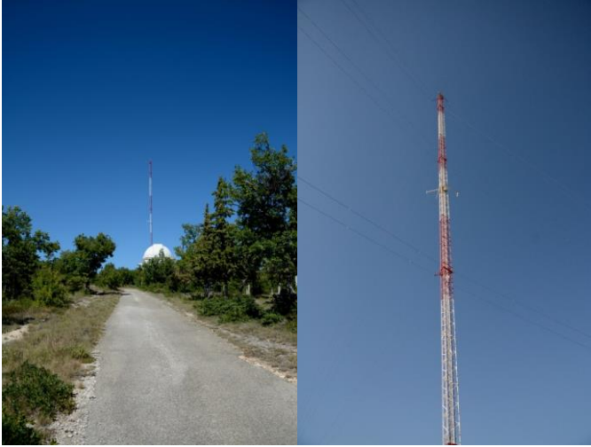
Fig. 4: The ICOS tower at the OHP site.
