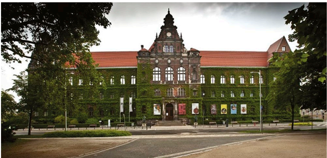
Figure 38. The front of the Main Building of the National Museum Wrocław.
