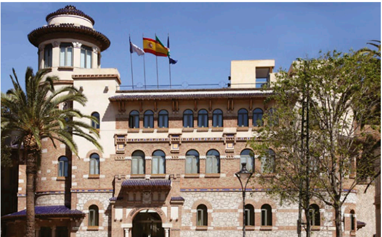
Figure 4. The Rectorate Building in Malaga (University of Malaga).
