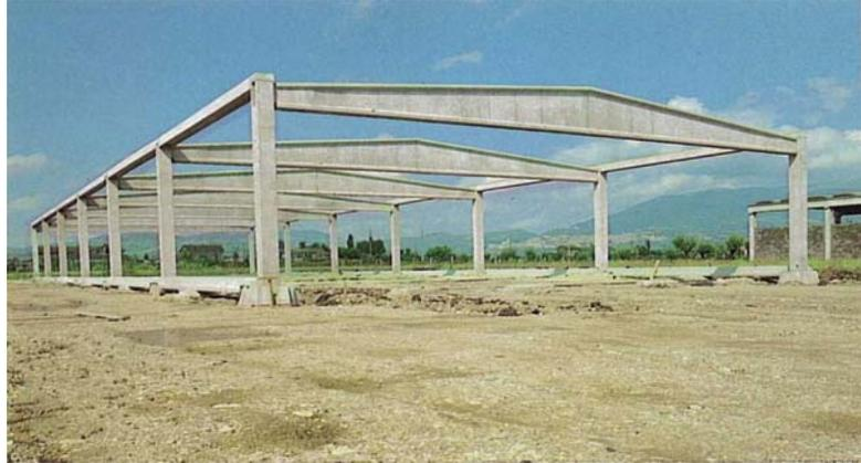
**Figure 2:** precast structure of industrial building
