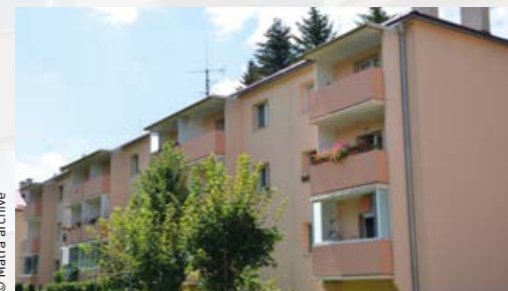
Renovated and modernised building
