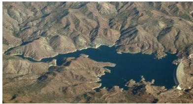
ET9.2: Artificial reservoir with dam infrastructure, Cyprus.
