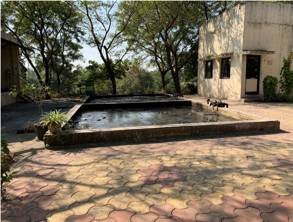
Sludge drying beds
