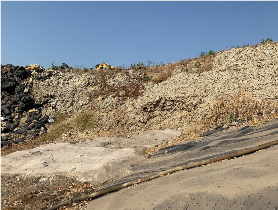
Landfill Cell 4.1: Hazardous waste cell
