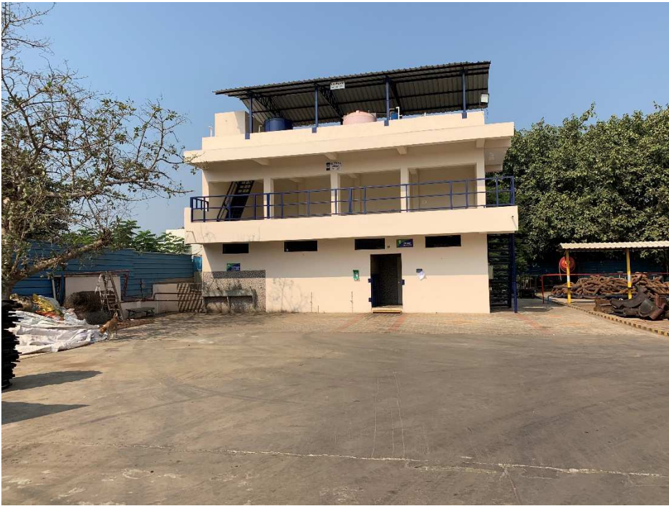
New workers facility with toilets, showers and shaded rest area.
