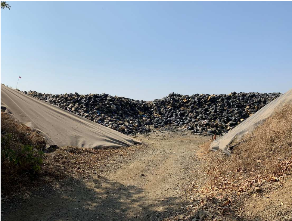
Landfill Cell 4.1: Hazardous waste cell
