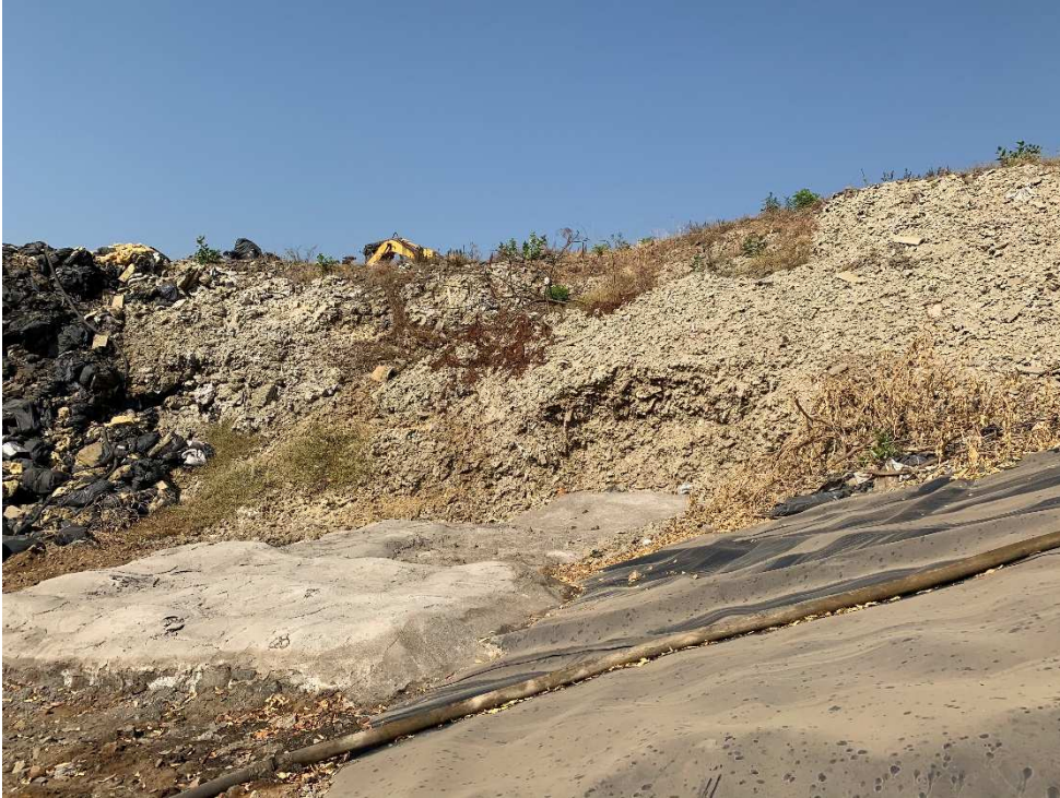
Landfill Cell 4.1: Hazardous waste cell
