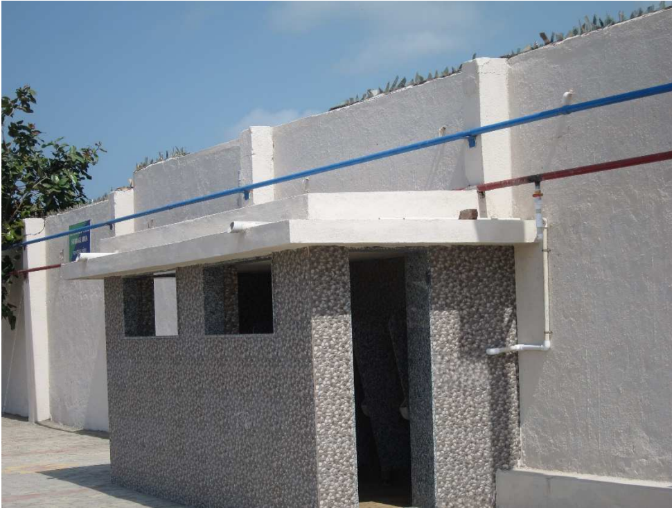
Toilets for workers.
