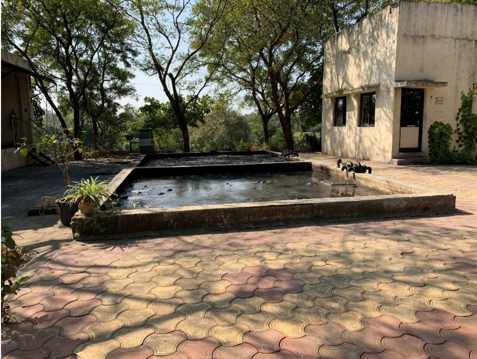
Sludge drying beds
