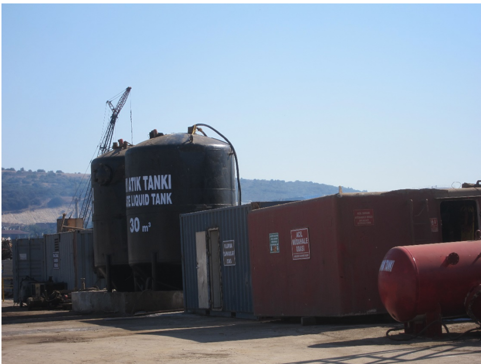
Water from the drain line is pumped into two tanks.
