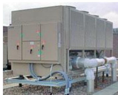
Chiller; source: www.acairsystems.co.uk
