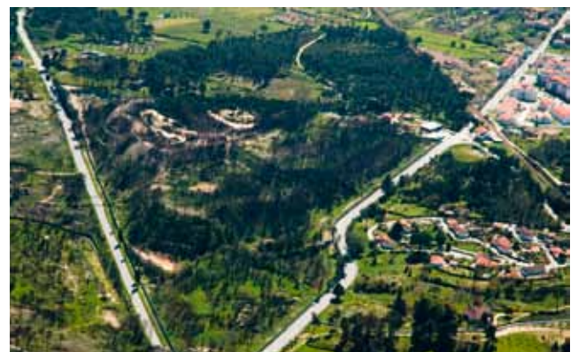
1 Old Dam after the forest fire occurred in the Summer of 2005
