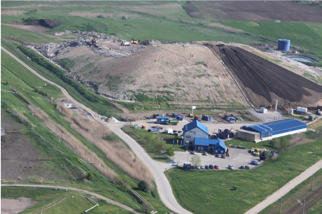
Figure 1.10-5: Overview of the non-hazardous landfill sites of A.S.A. (Romania)
