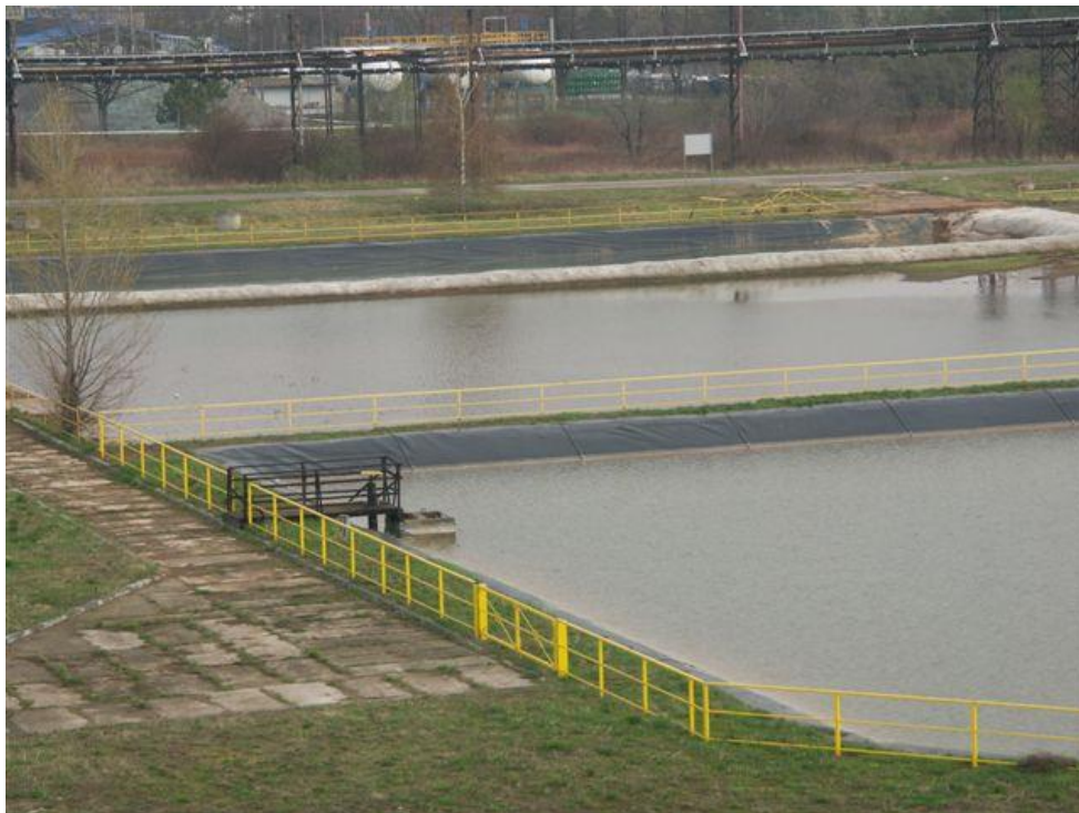
Figure 1.9-1: Landfill cell of Oleaon Eko Sp.z.o.o. (Poland)
