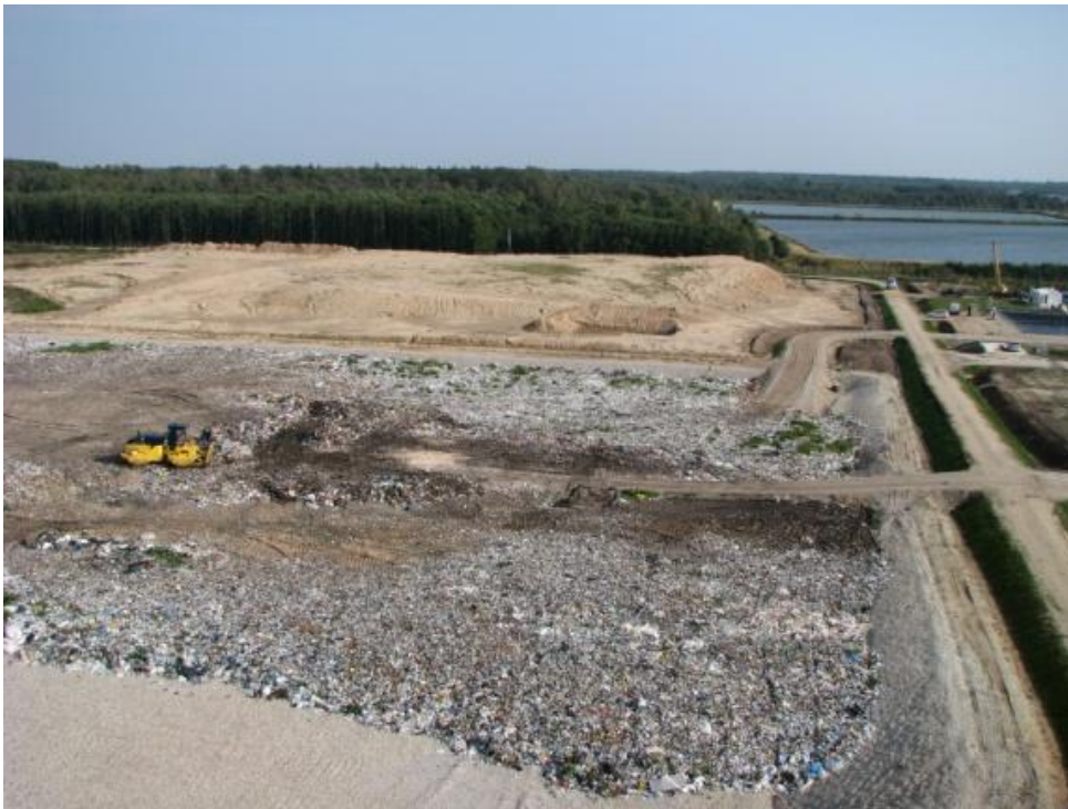
Figure 1.6-1: Overview of the non-hazardous landfill sites of Siauliai (Lithuania))
