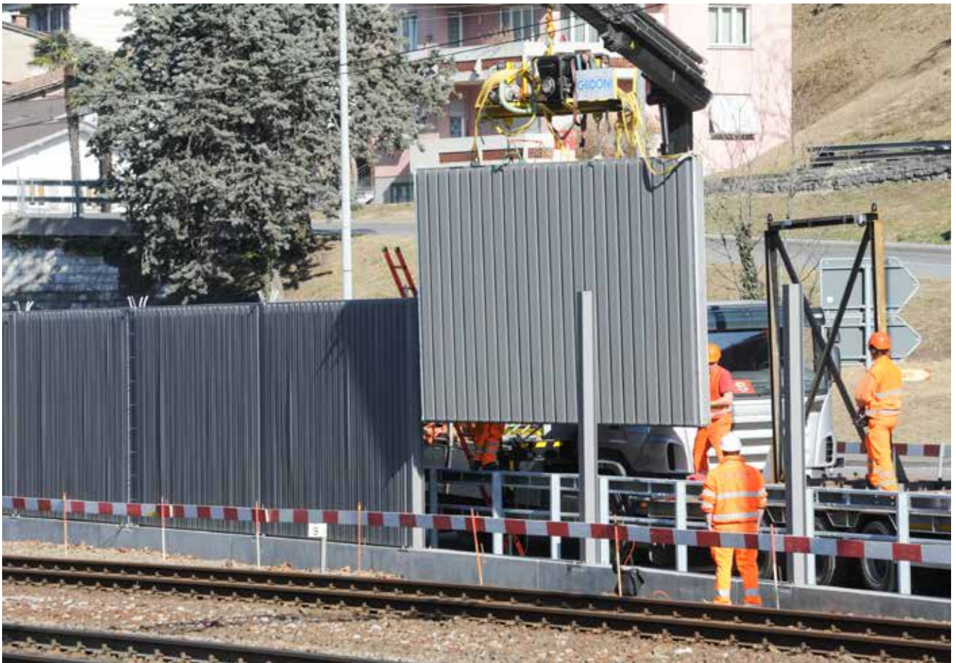
Workers during the installation of noise barriers on the railway. © istock / fotoember
