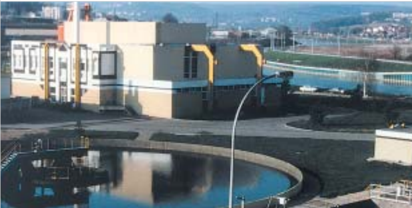
Waterbehandelingsinstallatie in Nancy.
