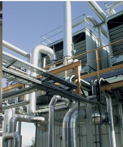
Left: new non-polluting and more efficient "dry" vacuum pumps.
