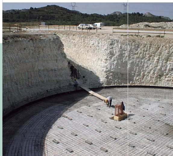
The NEPTUNE treatment plant under construction.
