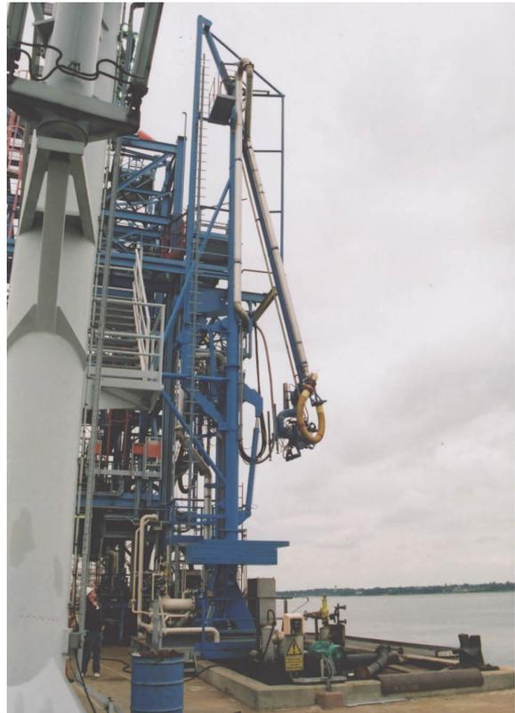
**Figure 10 - close-up of vapour return facility**
