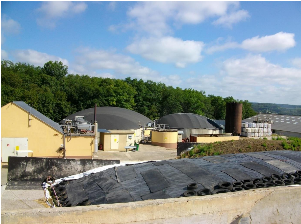
Faascht Farm: silos, eco-generation plant, digesters.
