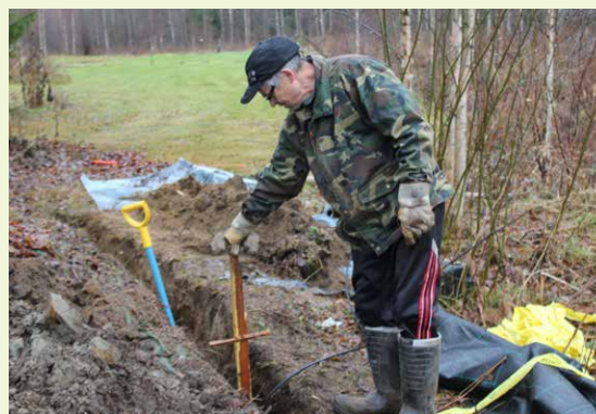
© Village Optical Fibre Network Cooperative of North-Western Kuhmo
