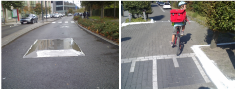
Cycle-friendly vertical and horizontal speed reduction (image source: D. Dufour)
