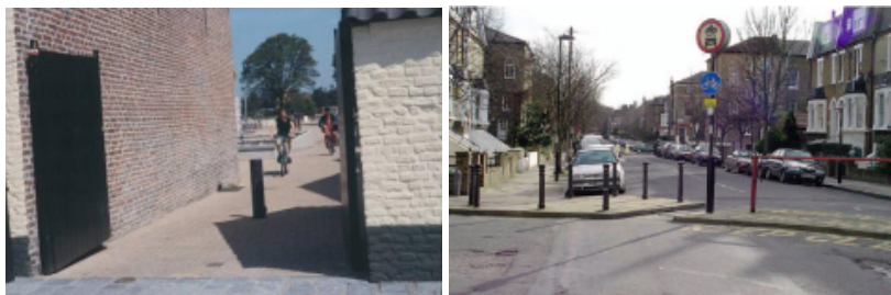
Road point closure with bollard or cycle bypass (image source: T. Asperges)
