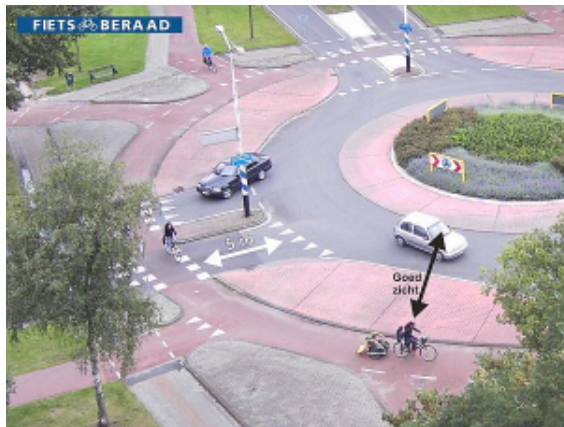
Single-lane roundabout with cycle track, with right of way for cyclists (Enschede, NL). Notice the typical circular design of the track and the colored crossings.
