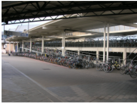
Multi-level bicycle parking at Ostend station (source: T. Asperges)
