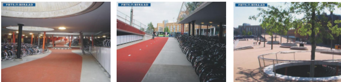
Interchange bicycle station at Groningen, underground, well-lit with daylight smooth access ramp (source: Fietsberaad – NL)
