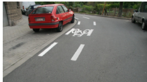
Advisory cycle lane to alert motorists of contra-flow cycling in a road bend, Brussels, BE (D. Dufour)
