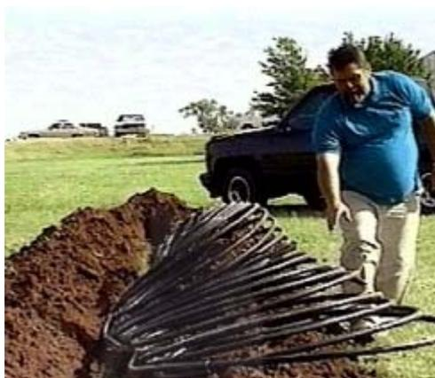
**Figure 3 Slinky-coil**
