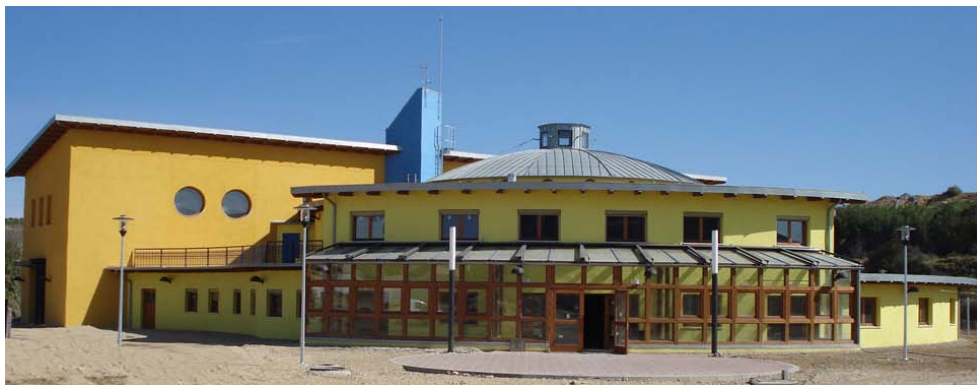
Figura 1.9. South current view of CIRCE Building.
