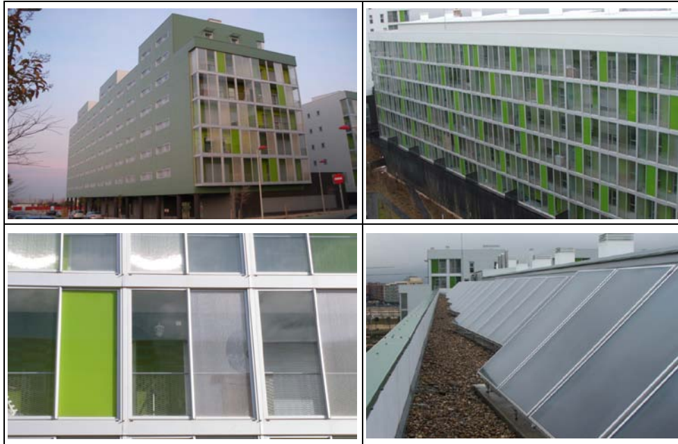
Figura 1.2. From left to right, up and down: North façade; South façade; Greenhouse detail; solar collectors on top of the roof.
