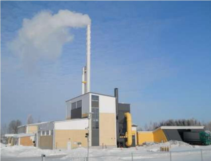
*Municipality heating plant equipped with a 10 MW<sub>th</sub> fluidised bed boiler and efficiency is enhanced by the recovery of the flue gas heat. Finland (Renowa Oy).*
