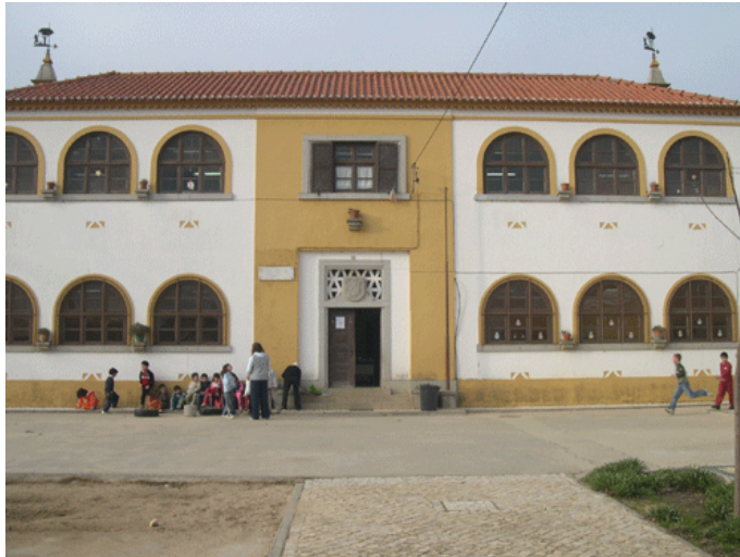
Figure 8-4: Primary school in Abrantes.
