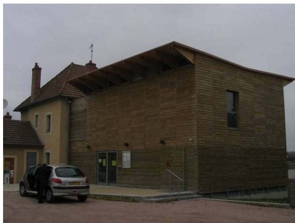
A vital meeting point – the Moulin des Roches at Toulon-sur-Arroux
