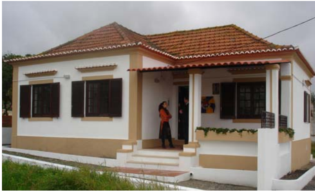
The house that will provide a centre for the DP's reconciliation activities
