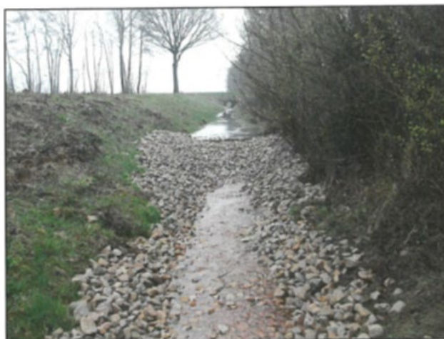
Figure 4: Lifted watercourse bottom in Germany
