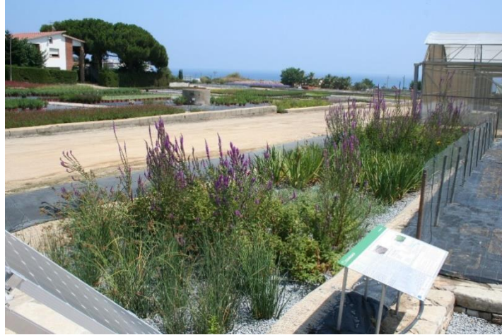
Figure 2 View of the constructed wetland, one of the techniques demonstrated in the CLEANLEACH® system at the Sala Graupera nursery (Sant Andreu de Llavanes, Barcelona-Spain).
